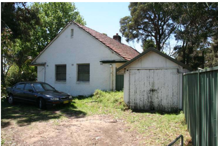
A Type D house with gable roof and free standing garage
