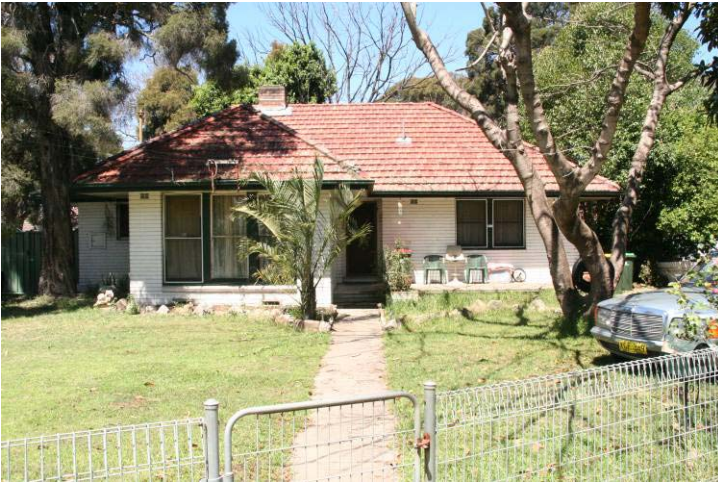
Type D house viewed from directly in front
