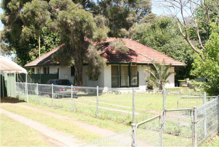
A Type D house, with hipped roof, viewed from the side
