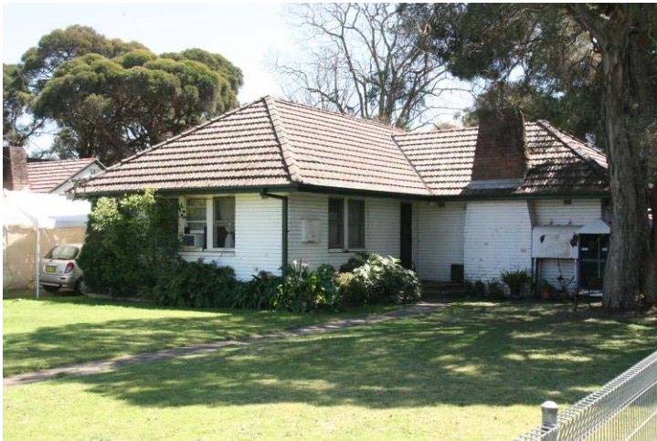
A Type A house with hipped front roof
